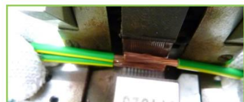
Figure 14. Correct positioning in the joint area for UCAB,[9]
